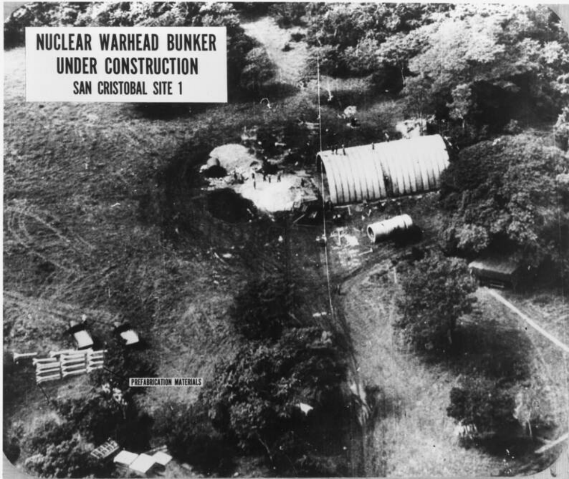
Department of Defense/National Archives A nuclear warhead bunker under construction in San Cristobal, Cuba during the Cuban Missile Crisis. October 1962.
